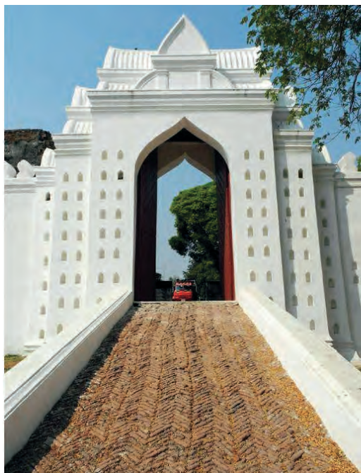
Figure 18. Fishtail brick road at Phra Narai Ratchaniwet, Lopburi
