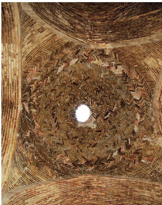
Figure 19. Fishtail brickwork on the dome of the central mosque, Isfahan
