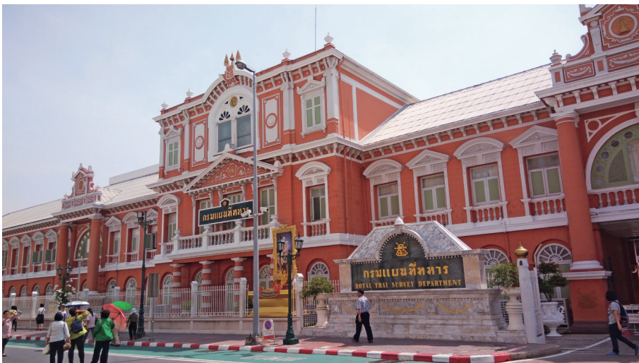
Figure 20. The Military College, redesigned by Cardu in 1889-91, today the Royal Thai Survey Department, Bangkok (Photo Koala0090)
