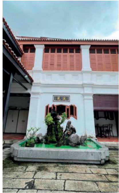
Figure 12. An air well, or open courtyard, in a shophouse in George Town, featuring granite slabs embedded in a recess to collect water. Source: Lim Gaik Siang
