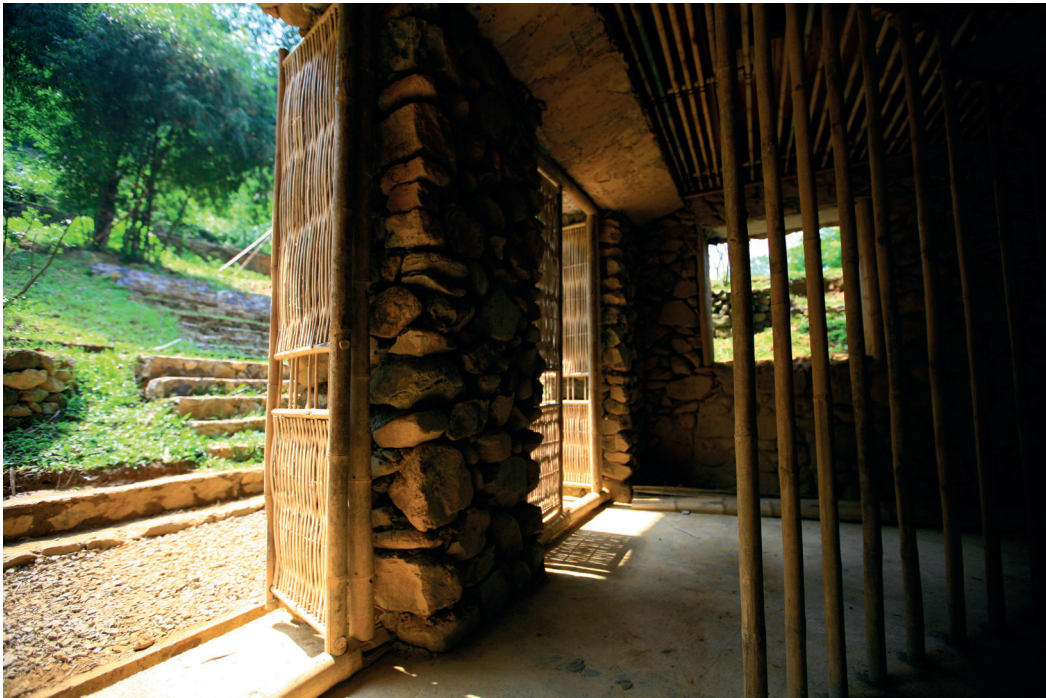
Figure 12. Natural stone and bamboo construction at Suoi Re Community House (photo: 1+1>2 Architects)
