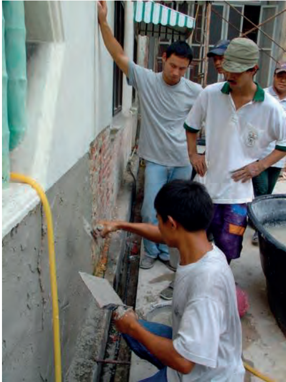
Figure 8. Stonemasons using lime plaster to repair an exterior wall in George Town. Source: Lim Gaik Siang
