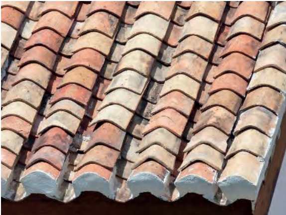
Figure 9. Terracotta clay U or V tiles on the roofscape of George Town. Source: Gwynn Jenkins and Tan Yeow Wooi, Introduction to Heritage Building Materials .
