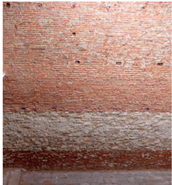
Figure 7. Exposed wall showing clay brick tiles in a shophouse in George Town. Source: Lim Gaik Siang
