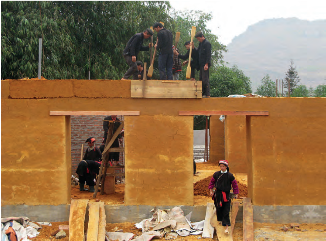
Figure 5. Rammed earth construction, Earth Village (photo: Son Vu / 1+1>2 Architects)
