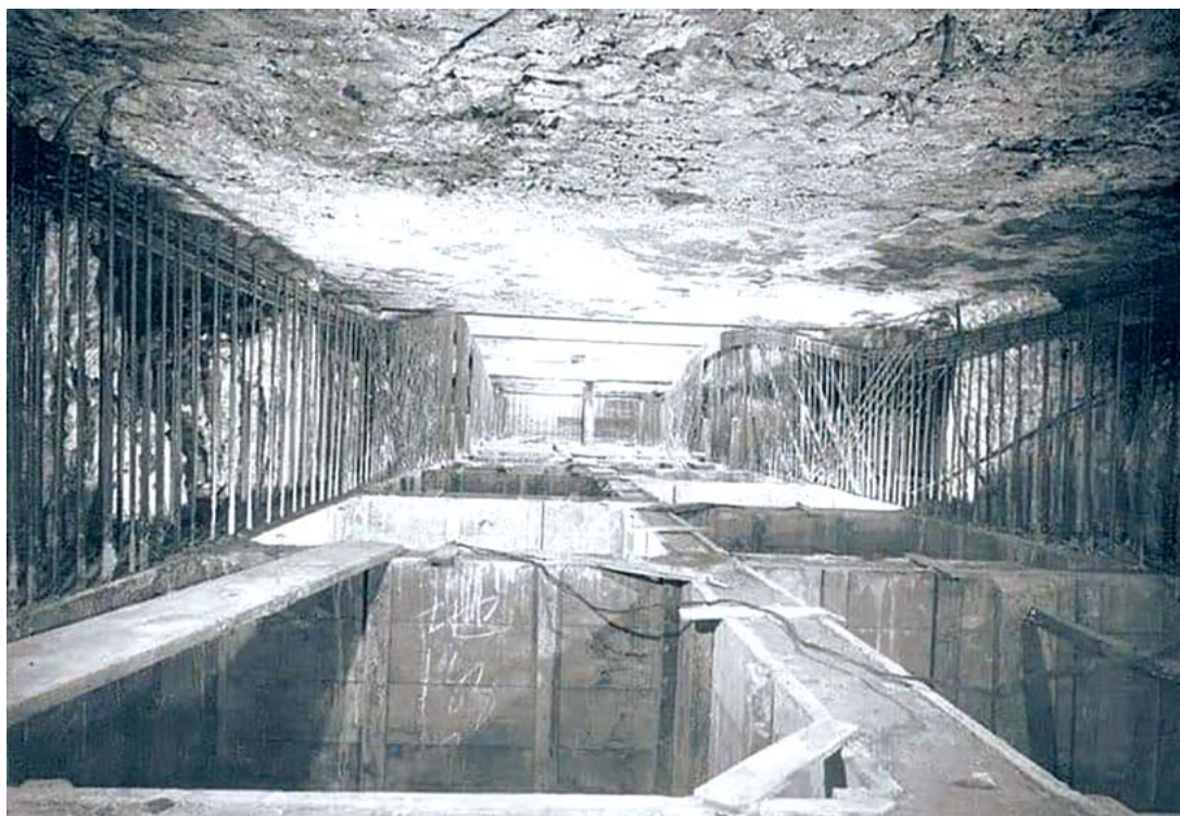
FIGURE 9: Photograph of the original foundation of the Ananta Samakhom Throne Hall during its conversion into caissons designed by Gollo, circa 1911 © NAT
