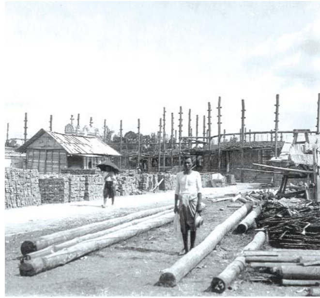
FIGURE 8: Brickwork at the Ananta Samakhom Throne Hall under construction, 1909, with scaffolding and stocked pressed bricks © NAT
